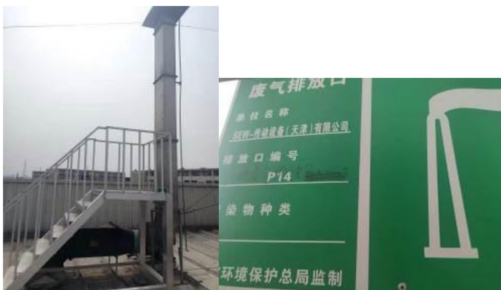
废液间废气排气筒 DA005
