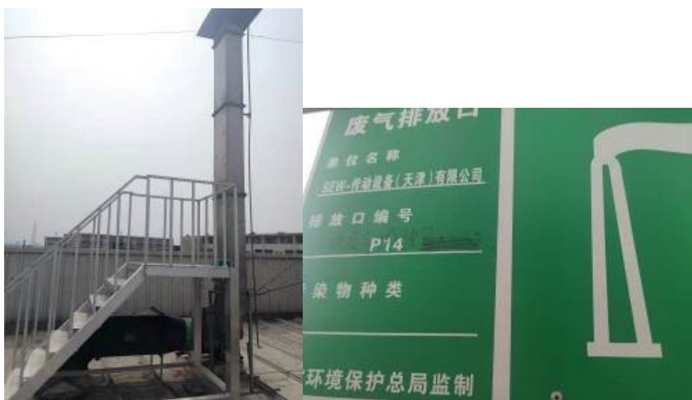
废液间废气排气筒 DA005
