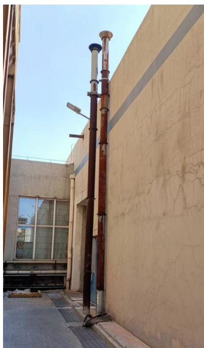
1#炭黑解包废气排气筒 DA001、2#炭黑解包废气排气筒 DA002
